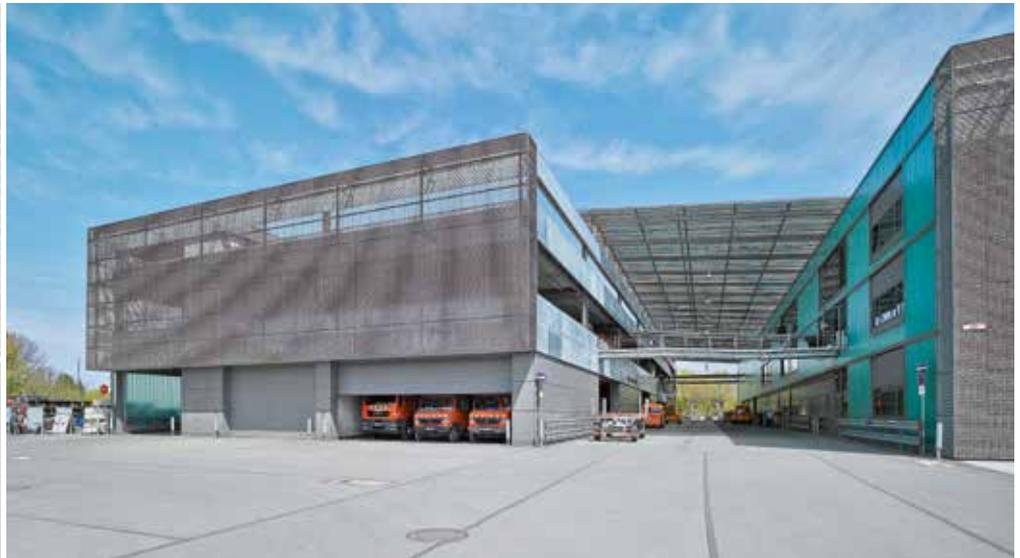
The fleet and storage rooms can be reached from within the covered walkway by means of industrial sectional doors. The inner rooms benefit from light falling into the walkway thanks to the glazing. (top)
