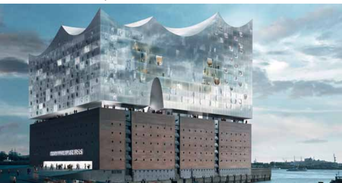
Elbphilharmonie under construction Architect: © Herzog & de Meuron, Basel, Switzerland
