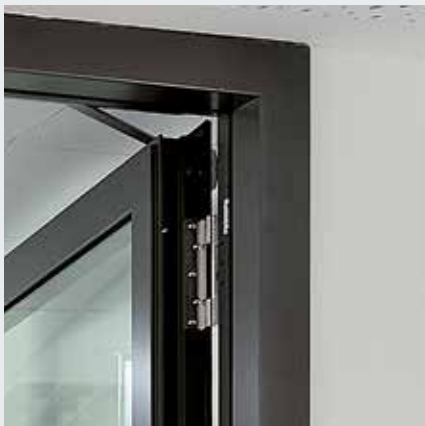
Frame prepared for overhead door closer
