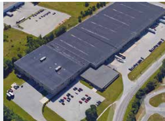
TNR Industrial Doors Barrie, Canada
